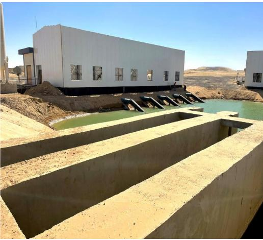
**Scope of Work:** Full Turnkey project for five water pumping stations and three HDPE water Pipelines Diameter up to 1200mm- 48 km length .
